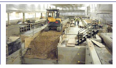
The construction of a new Weld S.R. pit (64m long x 9.5m wide x 2m deep) in the car assembly plant to facilitate the installation of a new robot weld line.
